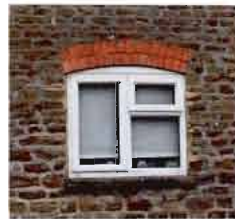
Example of arched redbrick lintel
