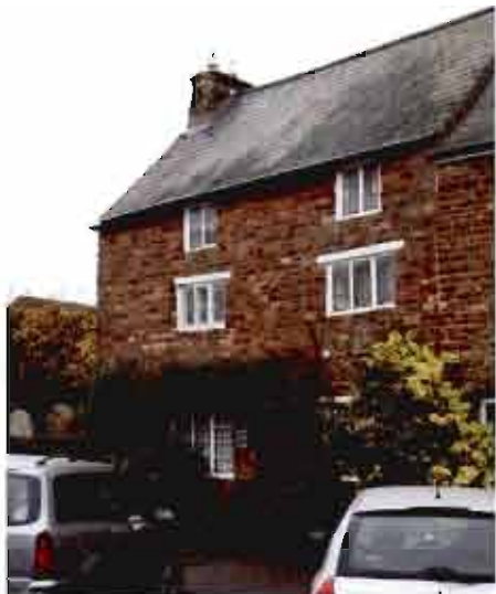
Example of 3 storey house in Dunston Ironstone, white timber lintels, grey slate roof
