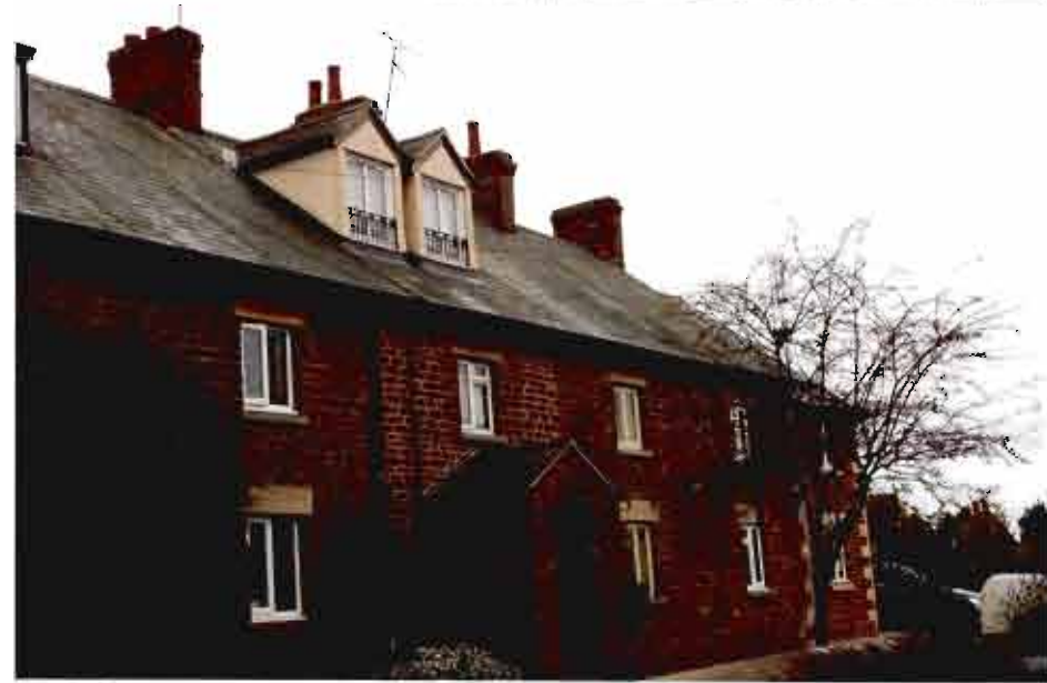
Example of rendered dormer window treatment on a cluster of cottages
