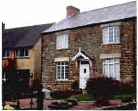
House in Dunston Ironstone with stone lintels, white painted timber pitched porch, note adjacent infill modern housing to left
