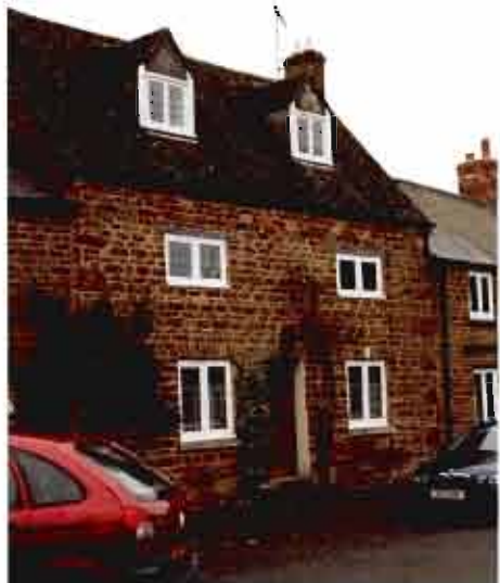
Example of 2 1/2 storey house in Dunston Ironstone, stone block lintels to ground floor, black painted timber to first floor, grey tiled roof, dormer windows to roof.
